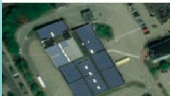
Busdepot Goslar 180 kWp, 2019
